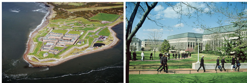
Figure 4. Views of (a) Fort George, north-east Scotland, from the air 18 , and (b) the US Naval Academy campus, north-east United States. 19
