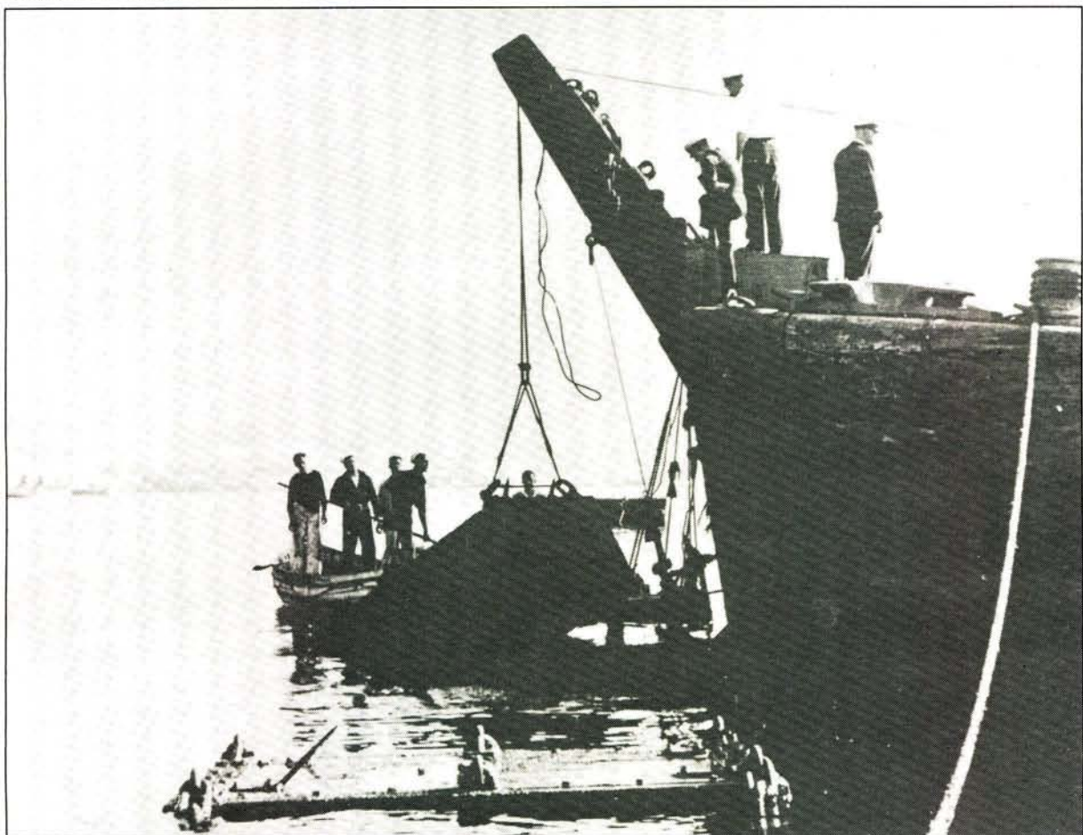
The mooring lighter lifting an anti-boat baulk at the harbour entrance in Simon's Town.
