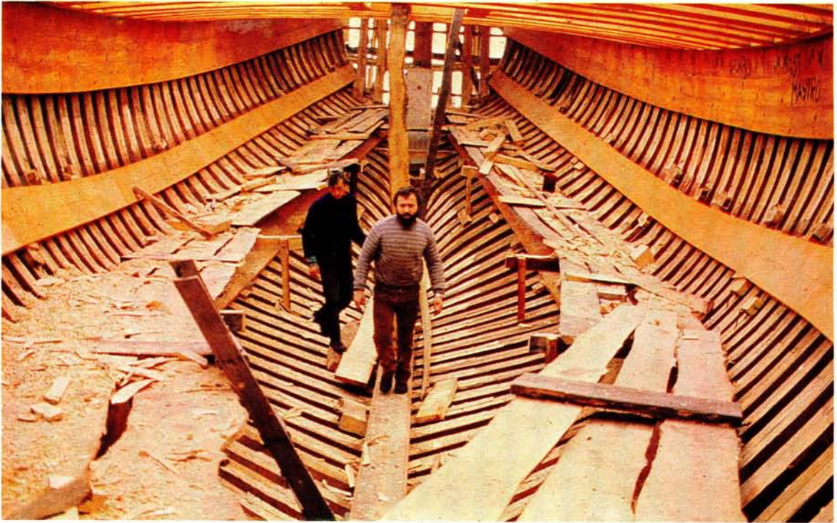
The replica caravel under construction in the shipyard of Samuel and Filhos in Vila do Conde near Oporto in Portugal. The vessel was designed by naval architects under the direction of Admiral Rogério S de Oliveira (Photograph: South African Panorama)
