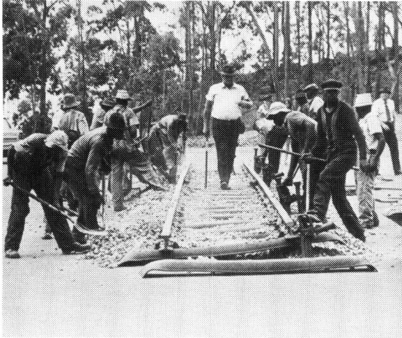
The construction of the Track
