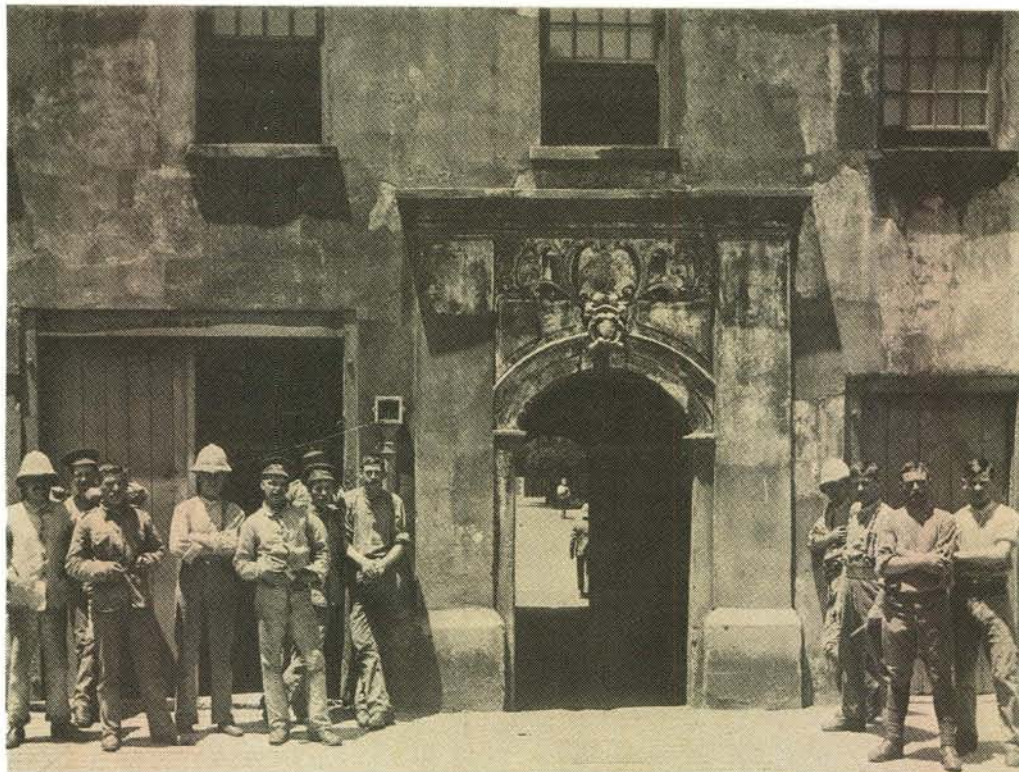
British Infantrymen outside the Sally Port between the Katzenellenbogen and Nassau bastions at the Castle. Notices above the doors on the left and right of the Sally Port indicate that these rooms were used for forage and groceries respectively.
