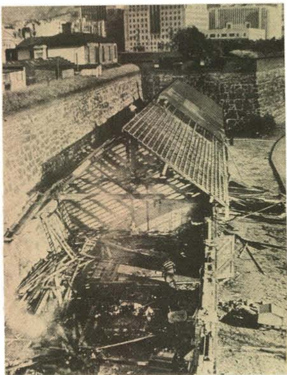
This photograph depicts the demolition of the wood and iron buildings between Katzenellenbogen and Buren on 2 August 1952.
