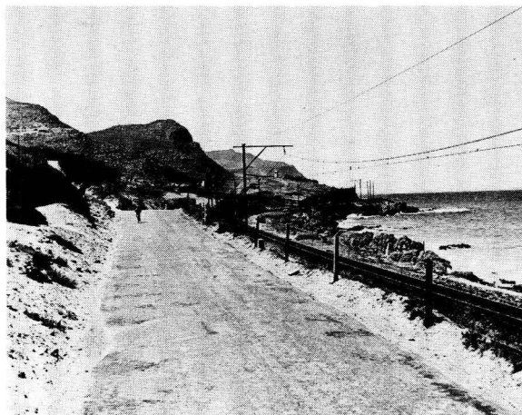
Lower North Battery seen from the main road from Simon's Town to Cape Town. Before the advent of the railway line, the road ran between the battery and the sea.
