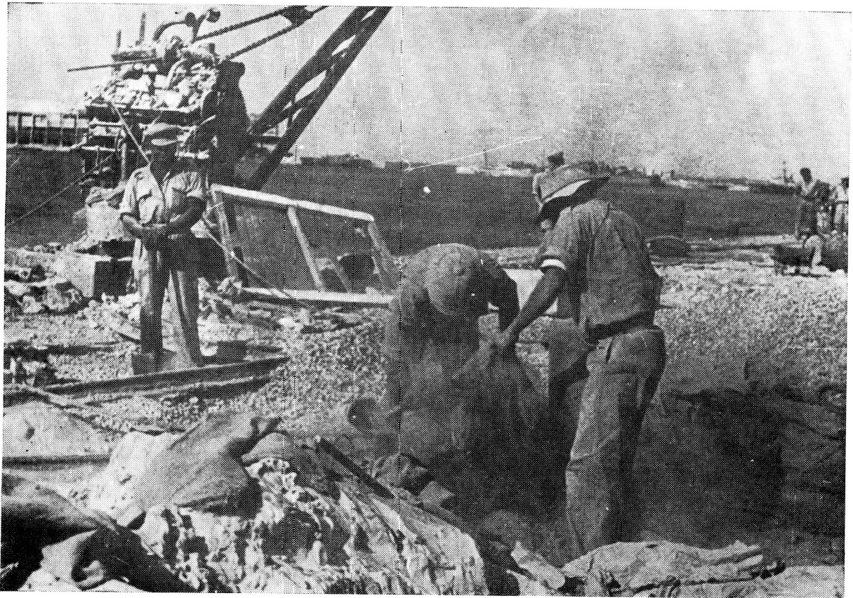
Sappers strengthening the coastal defences.
