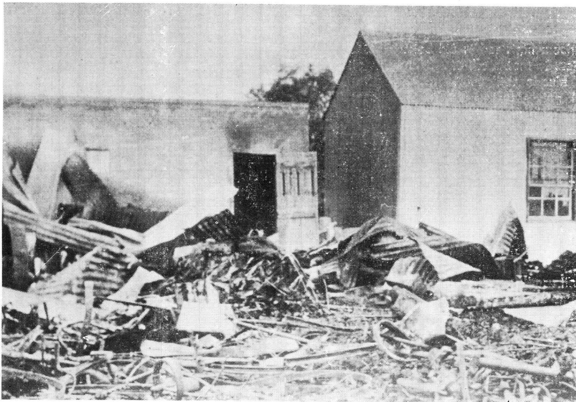
The charred remains of Weston's workshops, aeroplanes and threshing machine after the devastating Brandfort fire in February, 1913.
